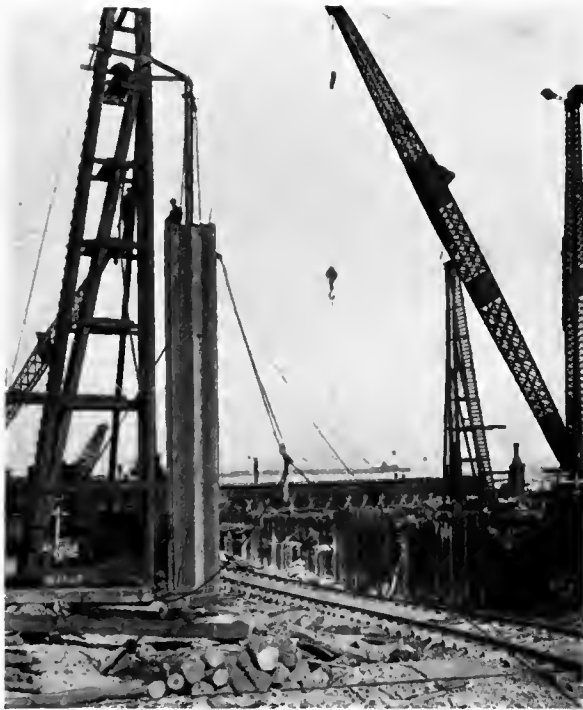
METHOD OF USING PILE DRIVER RIG Steel pipe holds cylinder of piling vertical for driving
